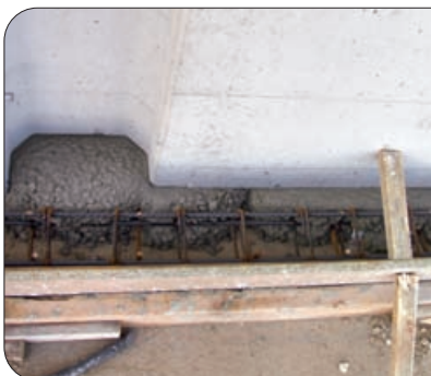
Concreting of perimeter reinforcement
