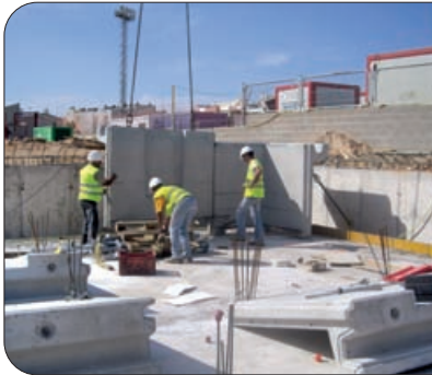
Fitting of the hydro-expansive cord
