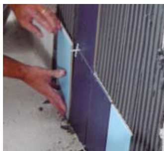
Set the slabs with TECNOCOL FLEX
