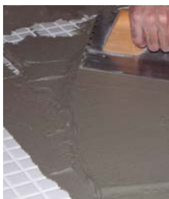
First layer of FIXMAX S2
