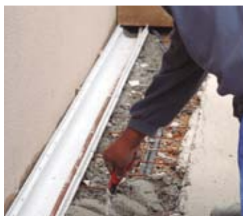
Placing the mortar around the channel
