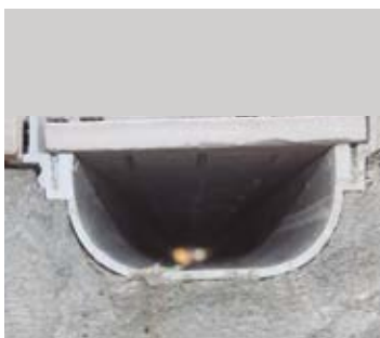
Detail of the channel embedded in mortar
