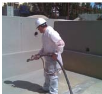
Application of HIDROELASTIC with a spray gun
