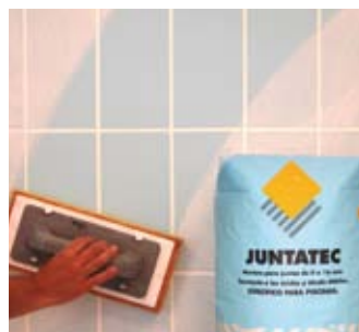
Grout using the special joint mortar for pools JUNTATEC
