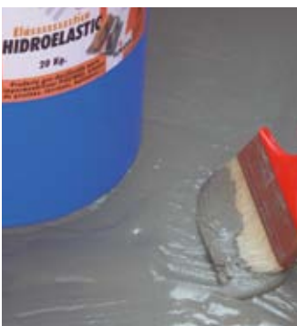
Application of HIDROELASTIC waterproofing
