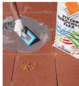
EUROCOLOR FLEX adapts to the joints from 0 to 16 mm
