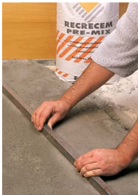
Applying the RECRECEM PRE-MIX screed mortar
