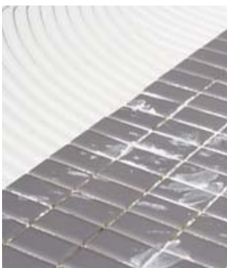
Lay the tile with FIXSET
