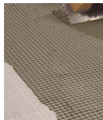
Covering the mesh with FIXMAX S2
