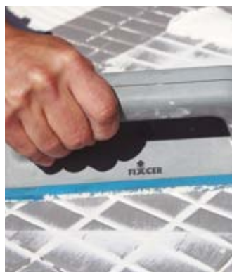
Grout the tile using FIXSET
