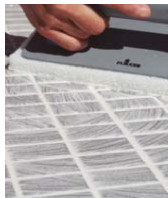
First clean with the trowel and then clean with a soft rag
