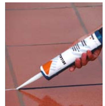
Fill in the expansion joints with SELLALASTIC
