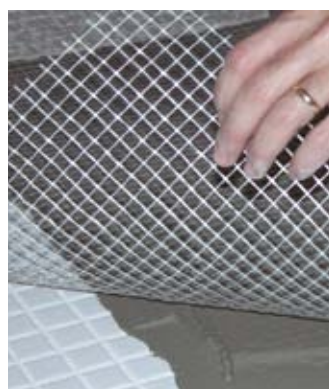
Placement of NET-MORTER-110 mesh
